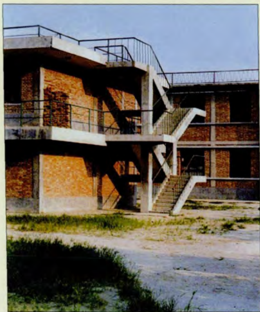
◆ 库区防汛避水楼
